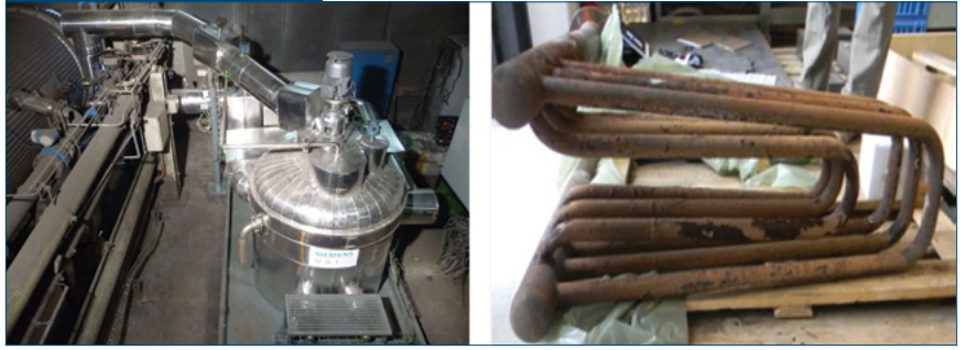
Heat recovery pilot plant at a steel plant in Germany.
