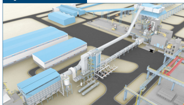
Waste heat recovery system for EAF.
