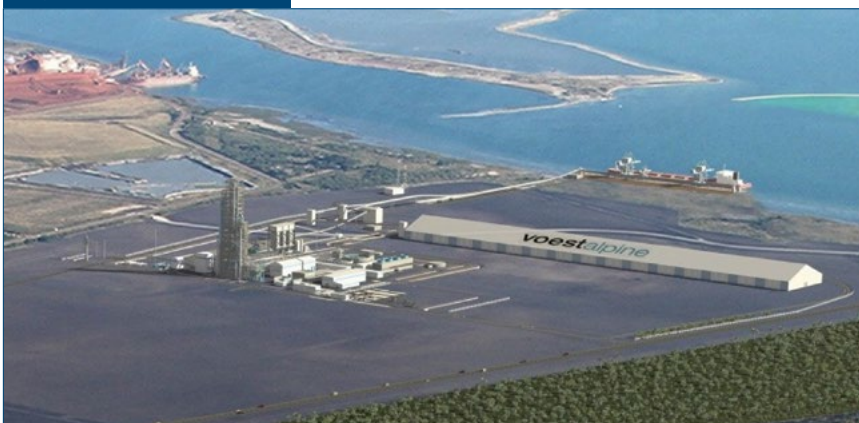
View of voestalpine Texas LLC HBI plant site.
